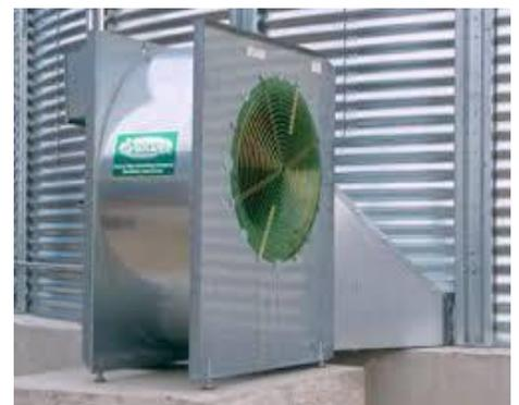
*Aeration Systems Installed to move fresh air through 30 Whole Food Storage Silos*
